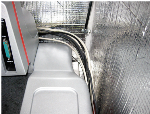
Figure 4.3k Rounded corner for cables
